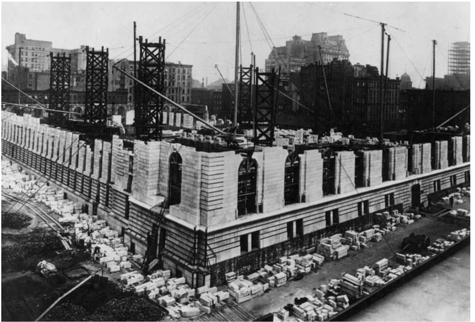
Under construction: the New York Public Library, 1902
