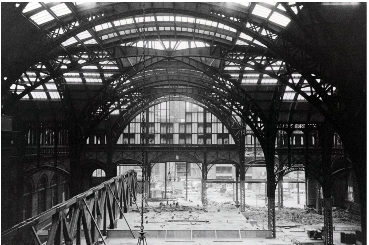
Penn Station during the demolition process, 1964
